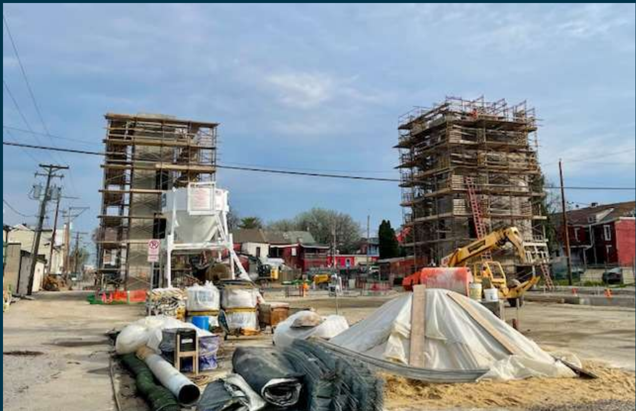
The Two Towers – The West and East Stairwell and Elevator Encasements
