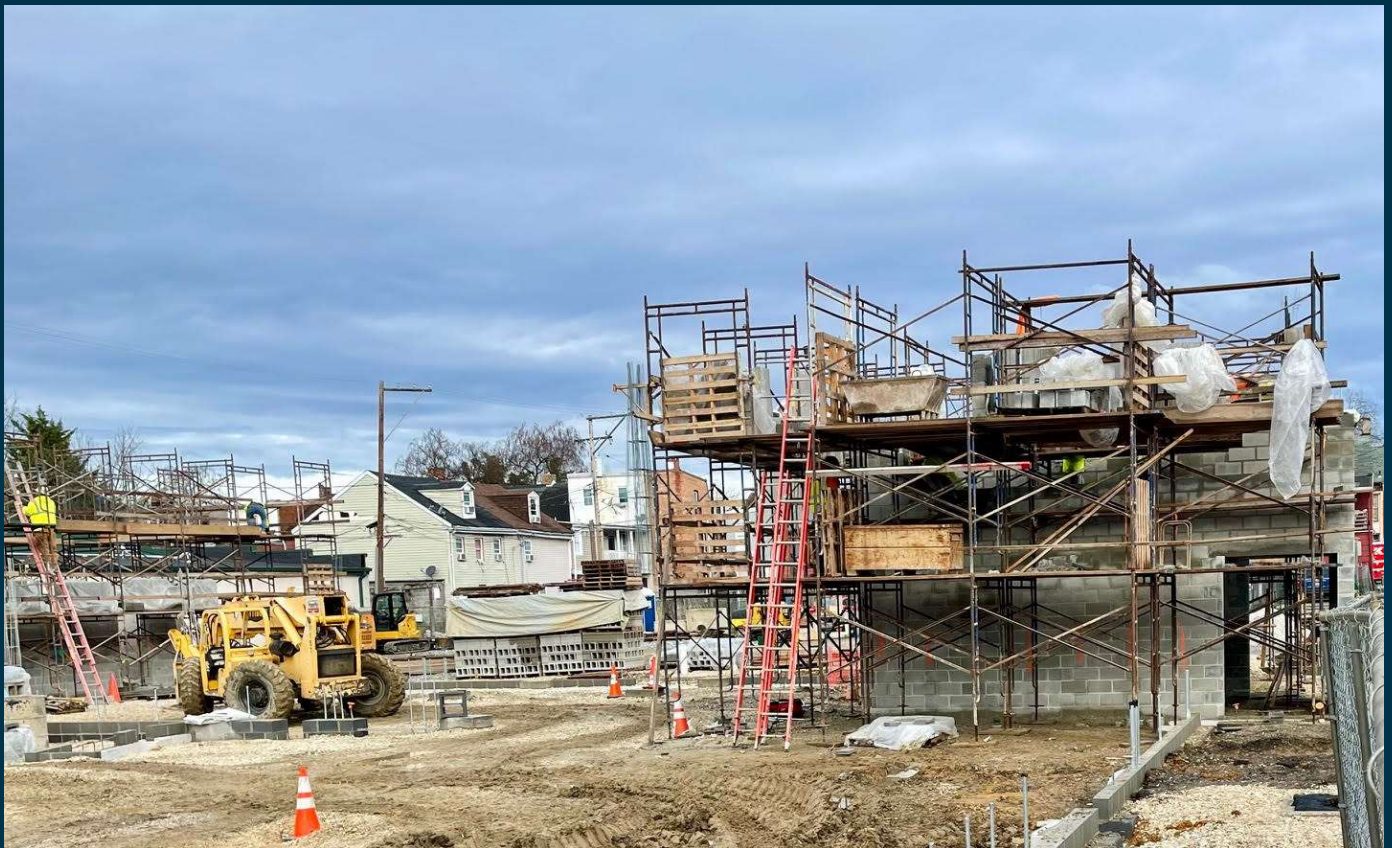
Photo shows scaffolding surrounding the East and West Stair towers
