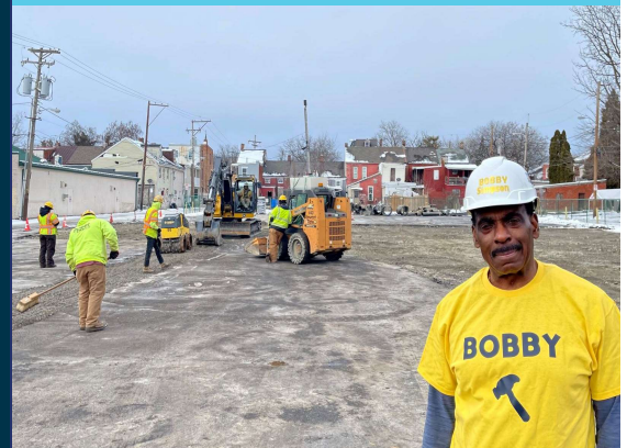
Bobby Simpson supervises site preparation for the HCC
